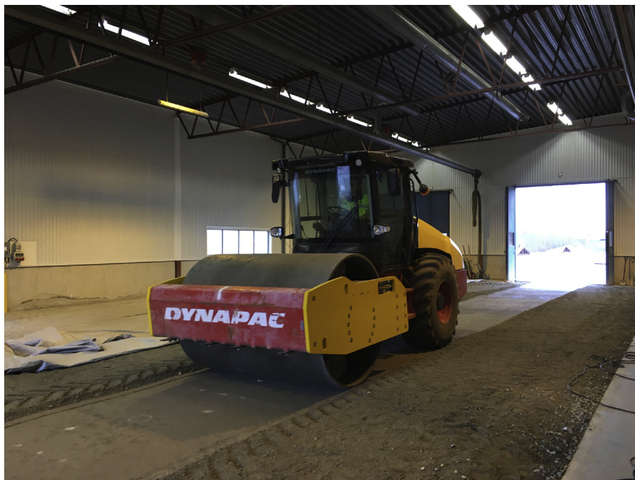
Fig. 1. Test bed and roller in operation.
