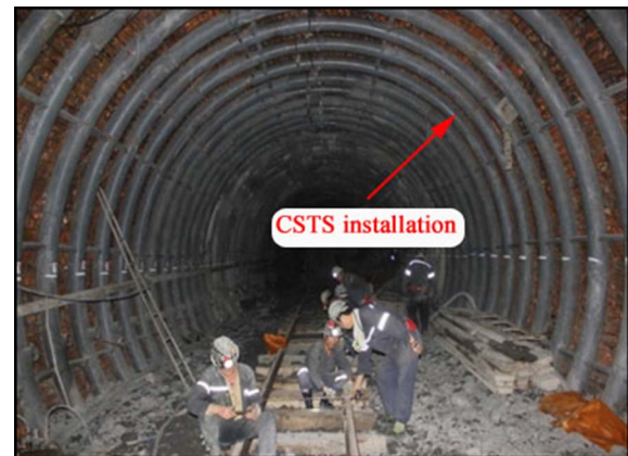
Fig. 3. CSTS installation inside a roadway.
