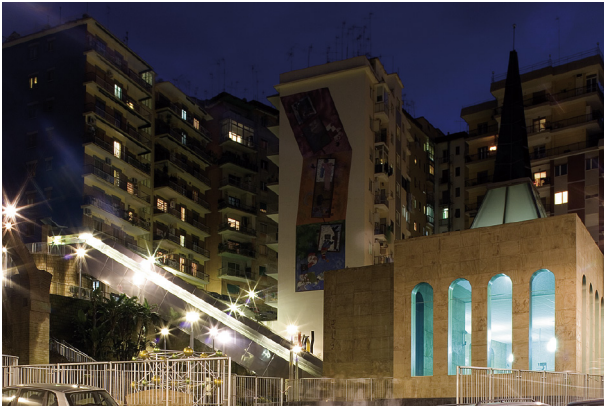
Fig. 1. Salvator Rosa Station. (Photo credit: Luca Pioltelli)
