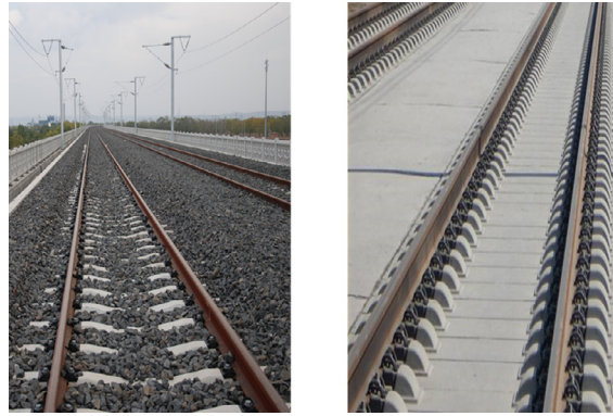
Fig. 1. Ballasted track and non-ballasted track.
