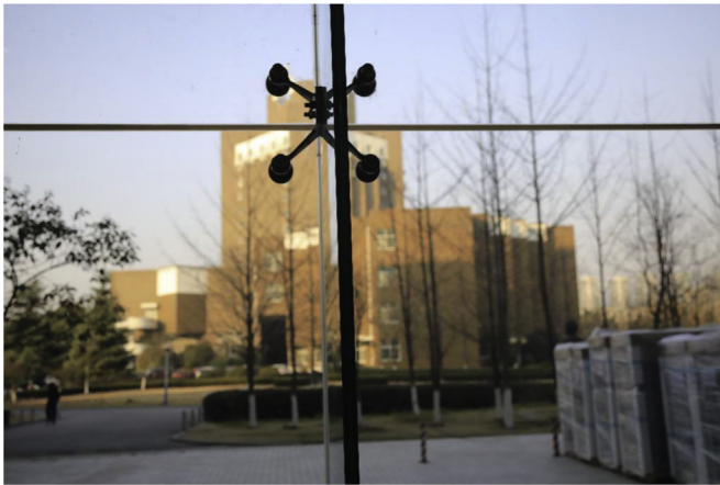
Fig. 1. Point-supported glass curtain wall, USTC campus, Hefei.
