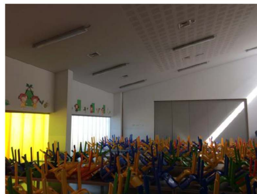
School AM - Ceiling (partial): perforated plasterboard with circular holes
