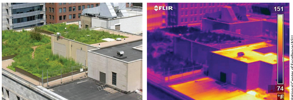
Fig. 1. Comparison of surface temperatures of a green roof and a concrete roof [5]. (For interpretation of the references to color in this figure legend, the reader is referred to the web version of this article.)
