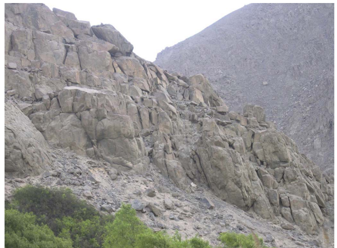
Fig. 1. Discontinuous rock slope damaged by the 2007 Pisco, Peru Earthquake.
