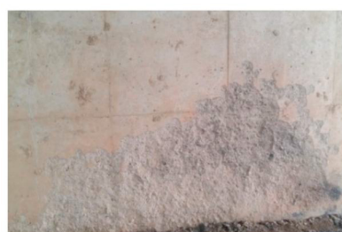
Fig. 3. Concrete damage
