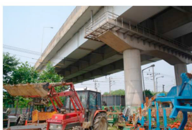
Fig. 2. High volt line under bridge
