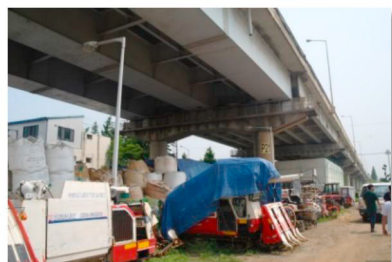
Fig. 1. Hazards under bridge
