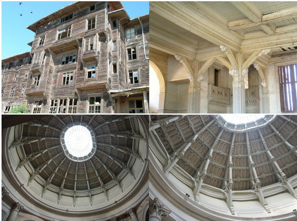
Fig. 1. Examples of heritage timber structures. Prinkipo Palace (Büyükkada, Turkey, 1903) – upper panel – Church of the Guardian Angels (Fermo, Italy, 1871. Arch. G. B. Carducci) – lower panel.
