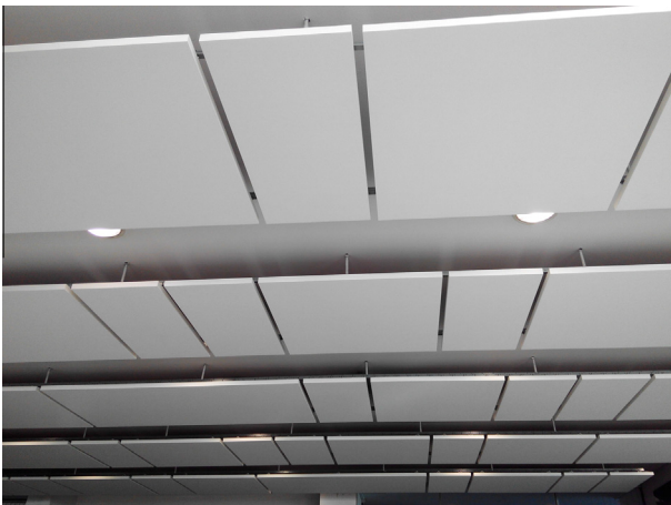
Fig. 1. Suspended ceiling with discontinuous absorbent material.
