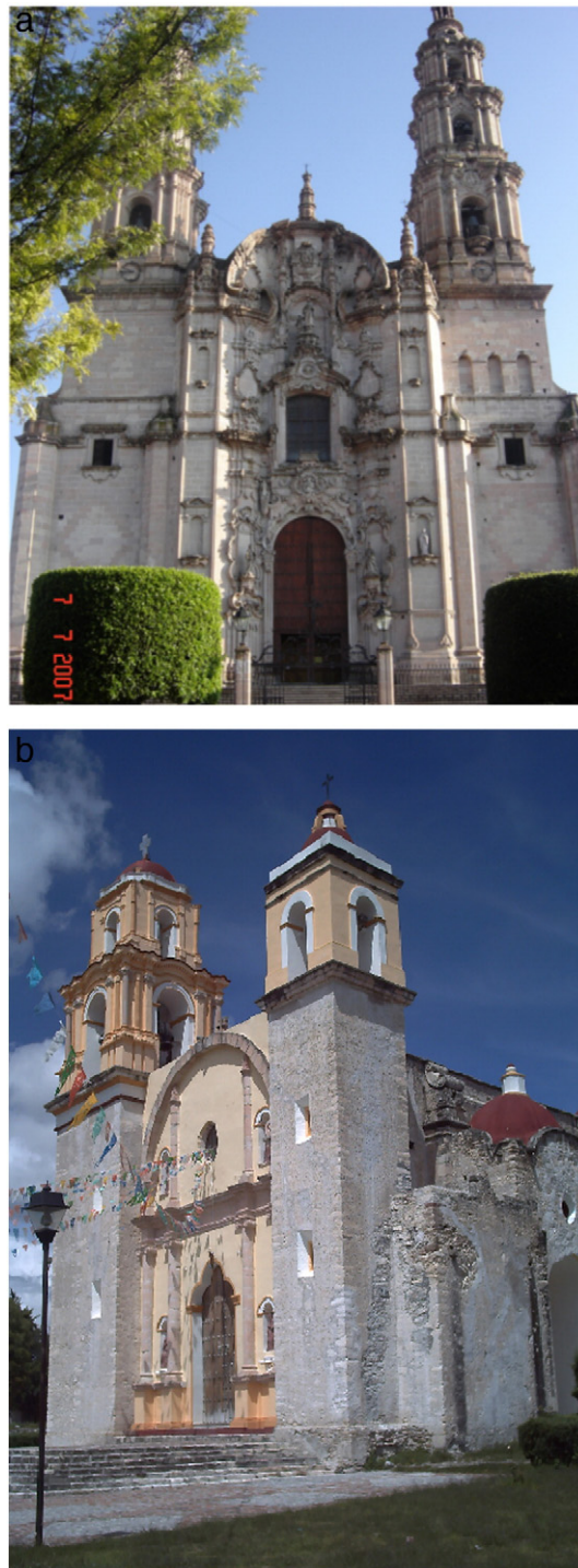
Fig. 1. Typical colonial churches built in: a) low seismic risk zone (central Mexico), b) high seismic risk zone (Pacific coast).
