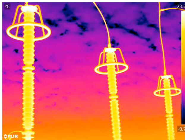
Fig. 1. A thermal image generated by a thermal infrared imaging camera
