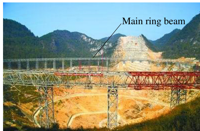
Fig. 2. Main ring beam of the FAST.
