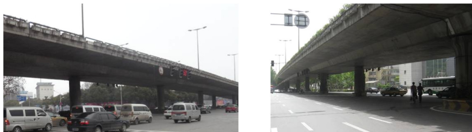
Fig. 1. Viaduct and its surrounding environment.
