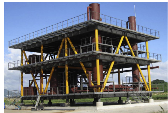
(a) Hypothetical FLNG topside structure at the KOSORI test site
