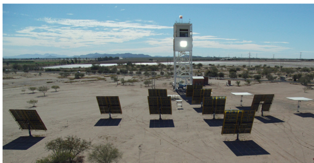
Fig. 1. Hermosillo's Solar Platform (PSH) – National Laboratory of CSP and Solar Chemistry Systems (LACYQS).
