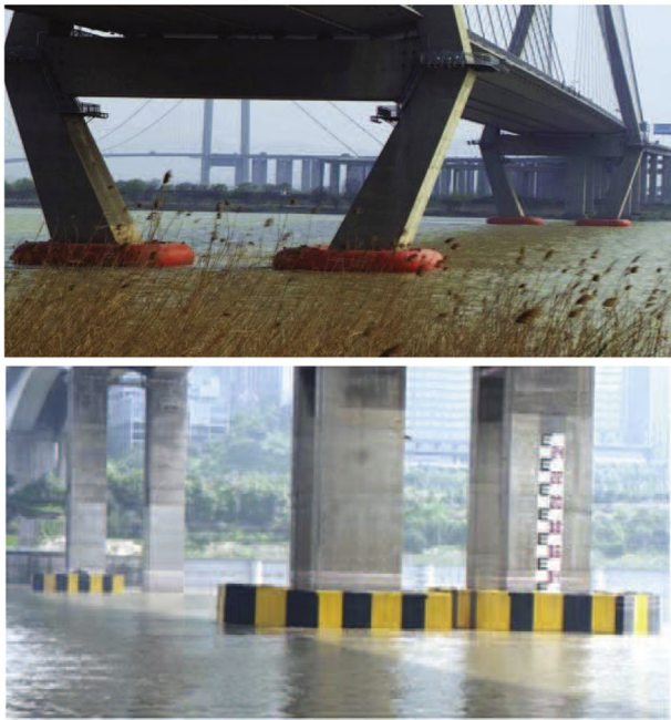
Fig. 1. Composite crashworthy devices installed for several bridges in China.
