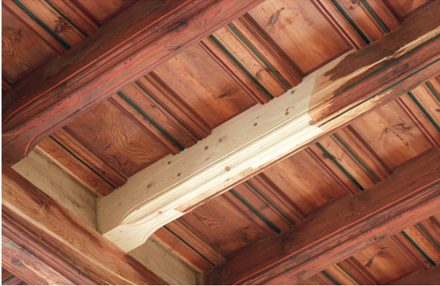
Fig. 1. Repair to a ceiling beam in Karlštejn castle dowel + 6 pins.
