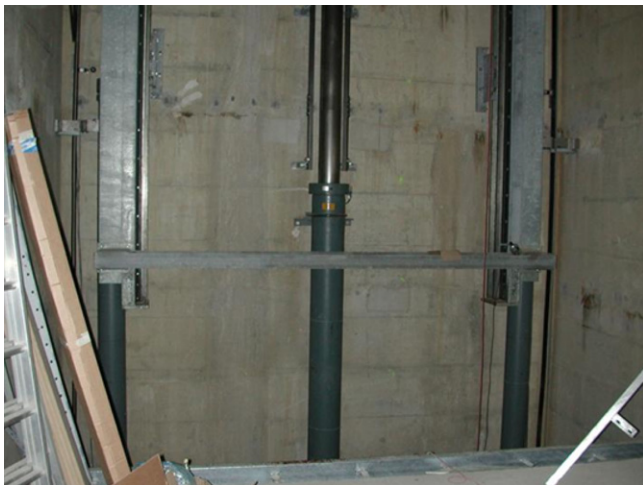
Fig. 2. Photograph demonstrating the electric hydraulics, so called piggyback-system. The middle hydraulic pillar was responsible for transporting the platform to an intermediate stop, where the platform is connected with the two other outside hydraulic pillars by bolts. Subsequently, the outside pillars transported the platform from the intermediate stop to the ground floor.
