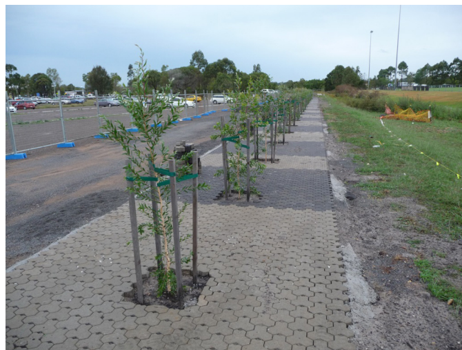
Fig. 1. Melaleuca quinquenervia trees immediately after planting in 3 m × 3 m permeable pavement plots between a car park and grass banking.
