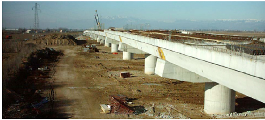
Fig. 1. Photo of Isola della Scala bridge during construction.
