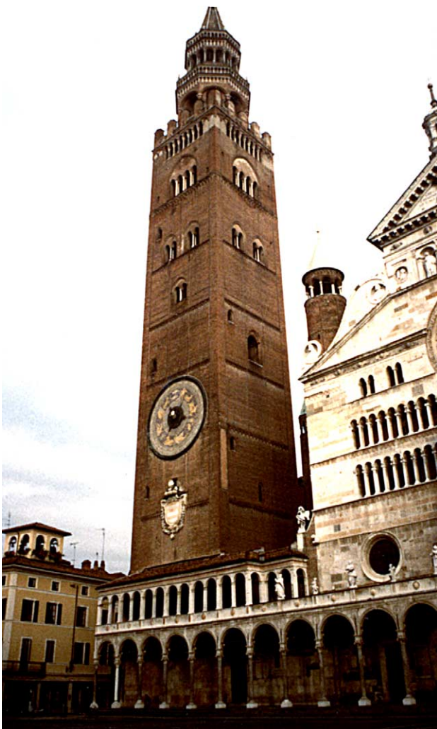
Fig. 1. Picture of the Bell Tower of Cremona (Torrazzo).
