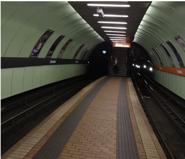
Fig. 2. A typical Glasgow Subway's platform.
