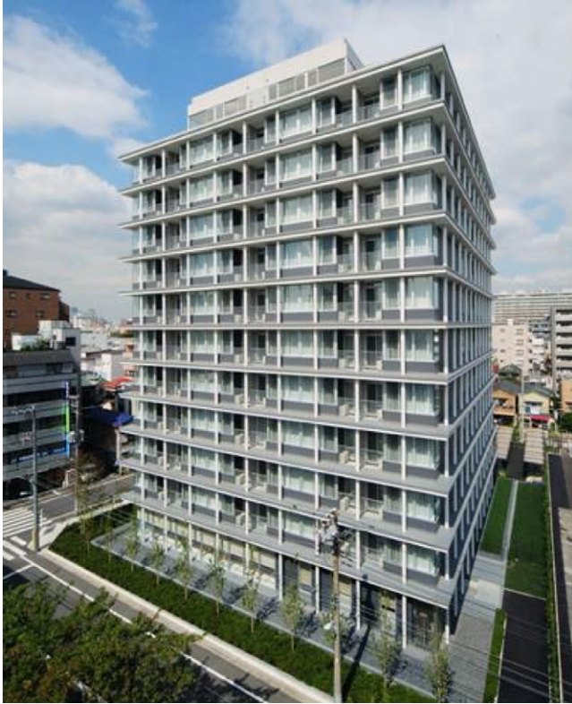
Photo 1. Twelve-story building in Tokyo.
