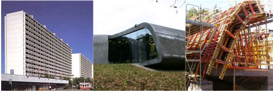
Fig. 1. Left: dominating geometry of today's urban landscape. Center: a prestige unique concrete structure. Right: handmade formwork for producing the unique concrete structure shown at the center photo.
