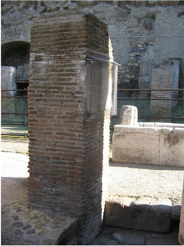
Fig. 1. The castellum aquae in ancient Herculaneum (Italy) near the crossing between IV cardo and decumanus maximus . The notice board, protected by a glass, is on the right of the pillar.
