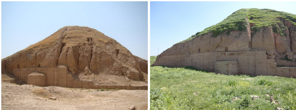
Fig. 2. Photos showing the state of burial of Al-Ziggurat walls at two different periods: 27 June 2011 (left), and 23 March 2013 (right).
