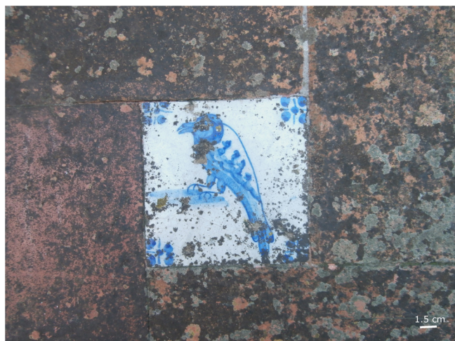
Fig. 1. Biological colonization of the unglazed and glazed ceramic elements of a garden bench situated in the historical centre of Sintra (Portugal).
