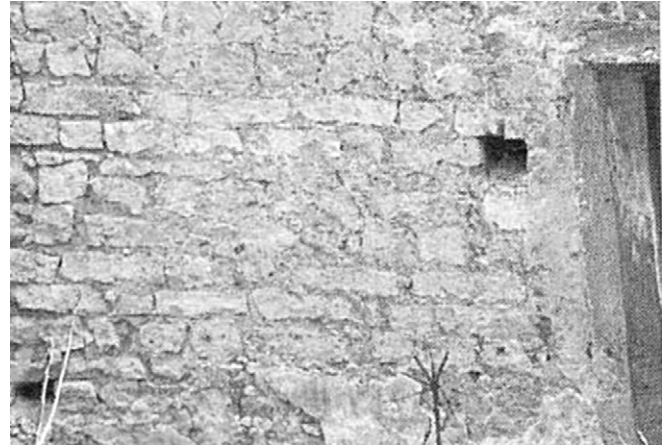
Fig. 1. Cantieri masonry wall ( S. Caterina a Formiello Church in Naples).
