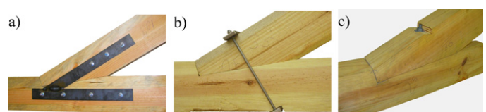
Fig. 3. Front notched connections with metal parts: a) bolted steel plates; b) external clamp; c) through bolt.
