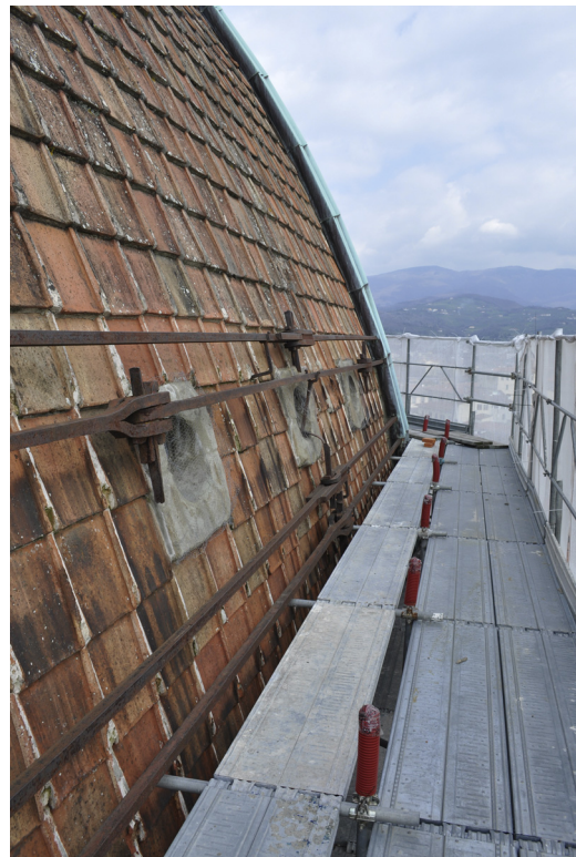
Fig. 2. Some orders of tie-rods on the dome.
