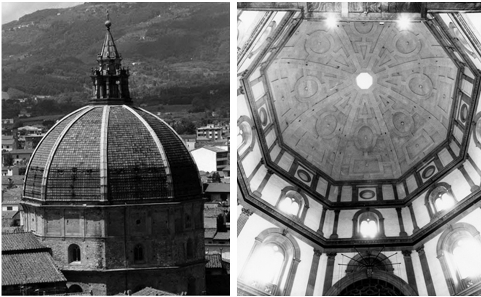
Fig. 1. The octagonal Dome; on the left, the seven orders of tie-rods are visible.
