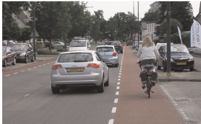
Fig. 2. On road bicycle lane along a distributor road.
