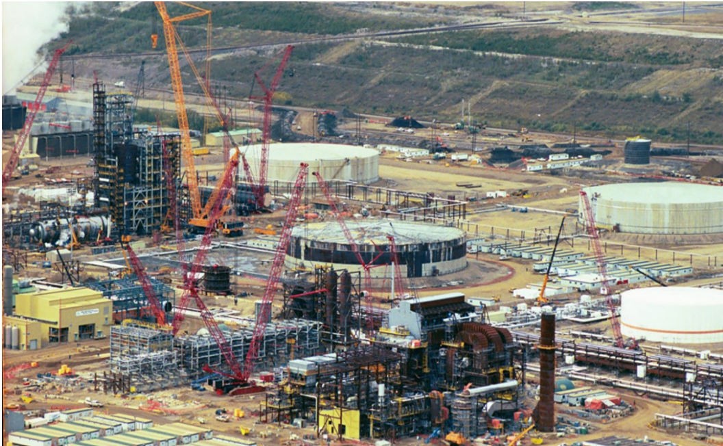
Fig. 1. Modular construction of an industrial plant.
