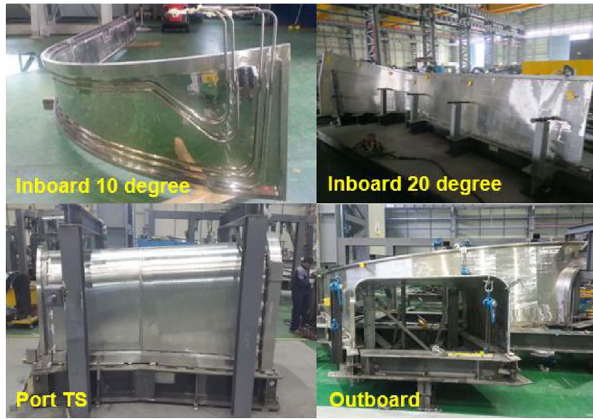
Fig. 2. Fabricated components of first delivery sector #6.
