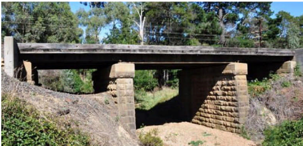
Fig. 1. Bridge 62 near Kilmore East, Victoria.
