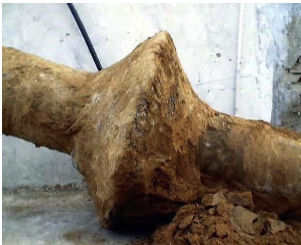
Fig. 2. Photo of excavated branch pile (Gao et al., 2009).
