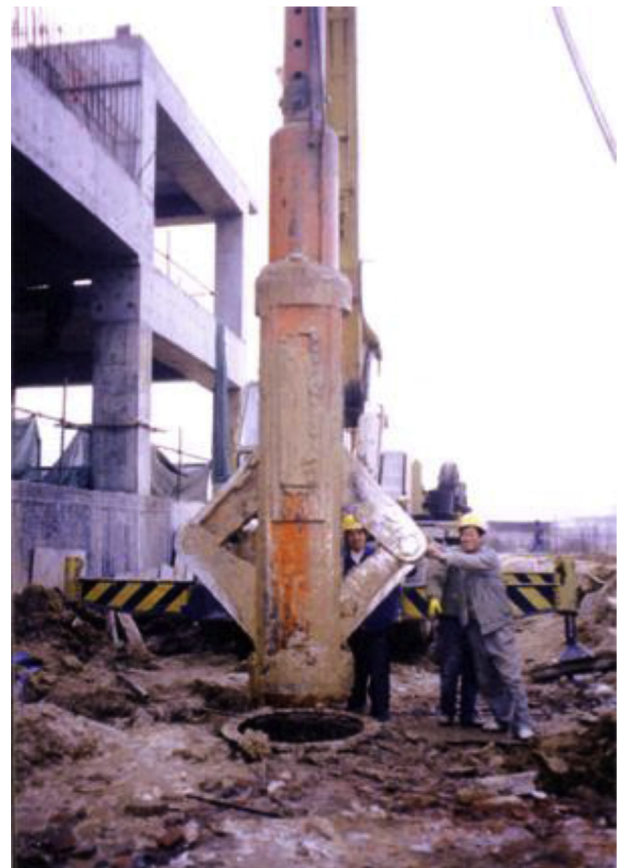
Fig. 3. Hydraulic squeezed machine.
