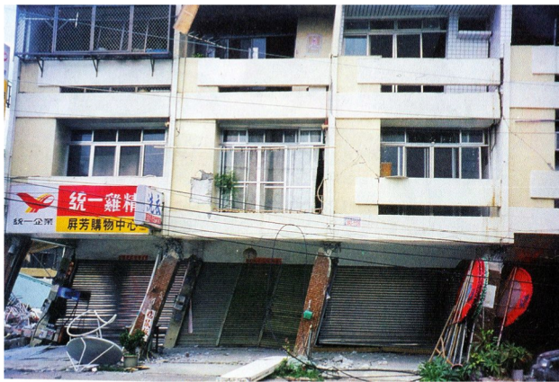
Fig. 2. Failure of the first story of row houses along the street direction during the 1999 Chi-Chi earthquake.
