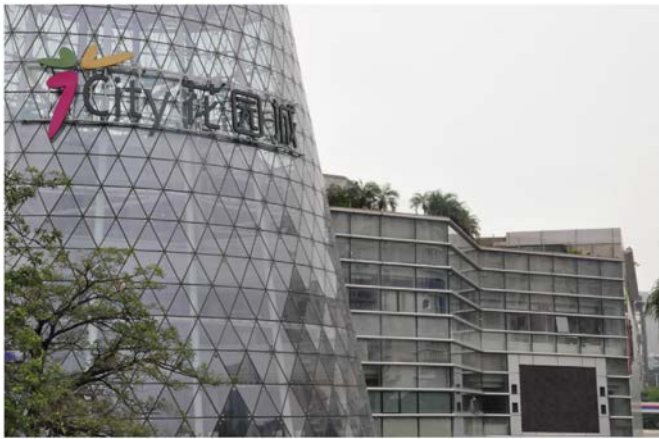
(a) Overall view of facade decoration
