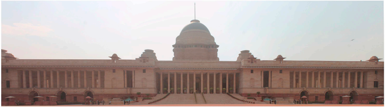
Fig. 1. The forecourt of the Rashtrapati Bhavan.
