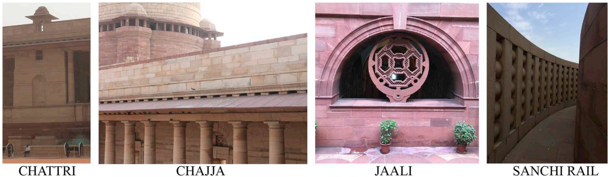
Fig. 2. Traditional Indian architectural elements in the structure- chattri, chajja, jaali and the Sanchi rail (from left to right).
