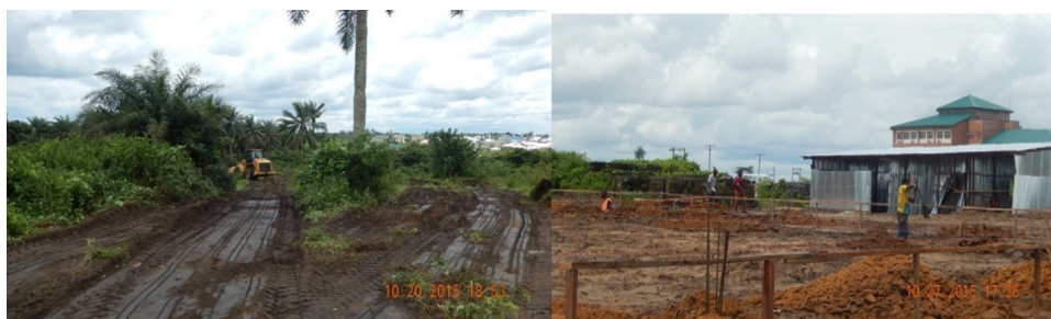
Plate 1. Land clearing of allocated site for the building.
