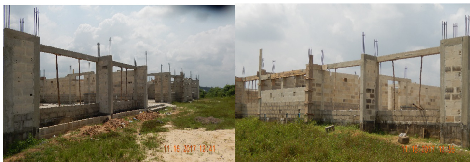
Plate 2. Current stage of the building.
