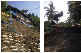
Fig. 1. the residential condition areas show 15% slope without any special treatment and unconsidered the mitigation aspect
