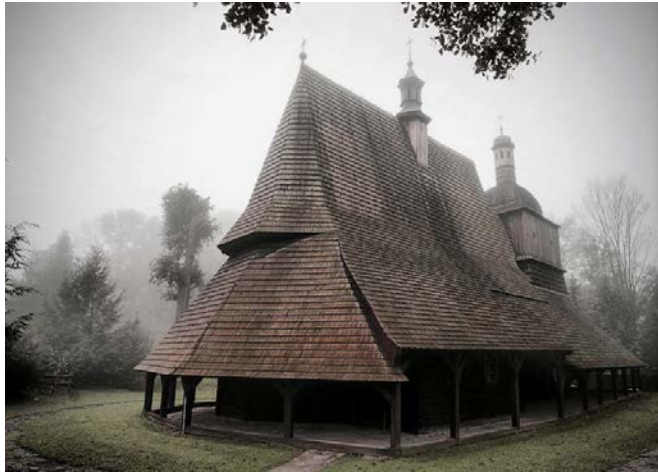
Photo 1 - The Catholic Church of Sts. Philip and St. James in Sękowa (Poland), wooden temple built around 1520, on the UNESCO World Heritage Site since 2003 (source: Fot. T. Tomaszek)
