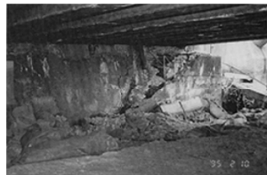
(b) A2 abutment
