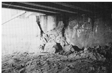
(a) A1 abutment
