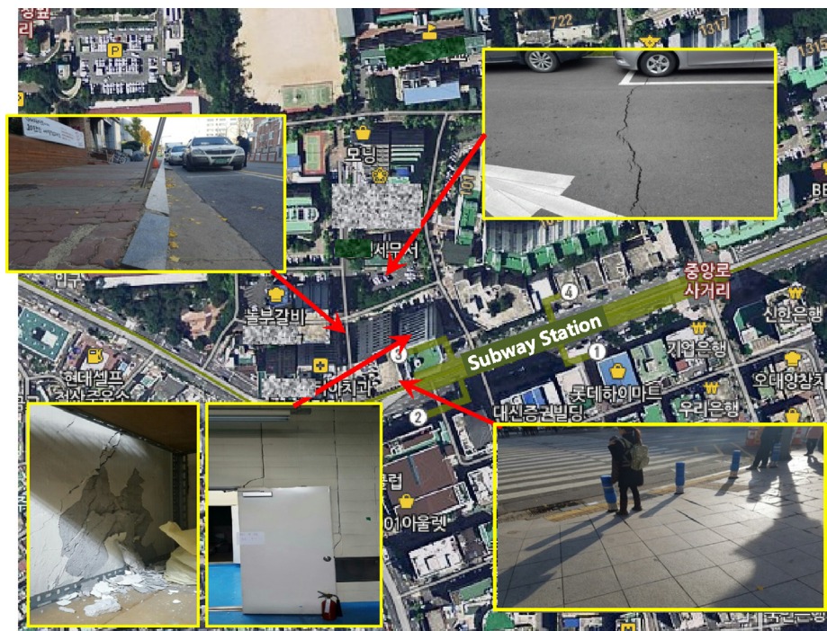
Fig. 1. Ground settlement due to excessive water inflow during tunneling.
