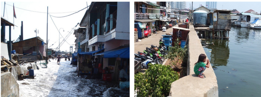
Fig. 1. Coastal town in Jakarta situated below sea level, which was extensively inundated during a high tide on November 26, 2007 (Left). The thin dyke protecting the settlement was raised by the local government by about a meter after the flood event, obstructing people's vision of the sea (Right). (Photo Left: courtesy of Brinkman J.J., Deltares - Jakarta flood hazard mapping 2007–2014, Right: taken by one of the authors on Sep. 2, 2015).
