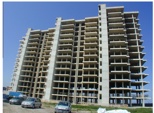
Fig. 2. Punta Perotti structure (Bari, Italy) before demolition.
