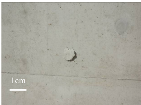
Fig. 1. Degradations induced by pop-out in concrete.
