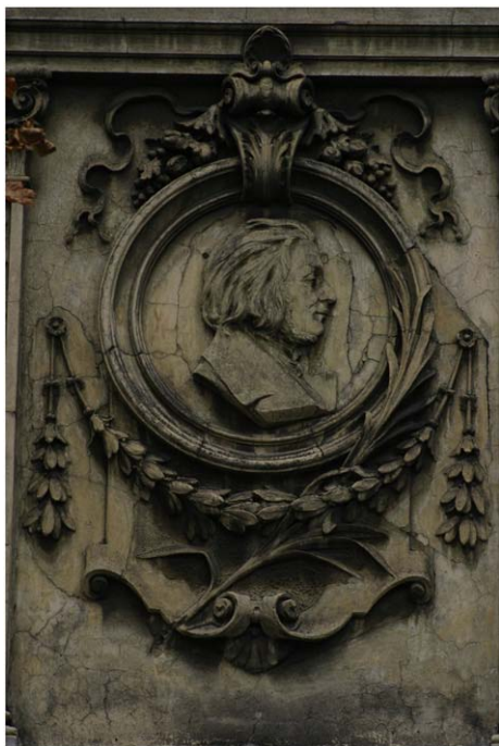
Fig. 1. Example of the use of Roman cement as a stucco and cast ornament.
