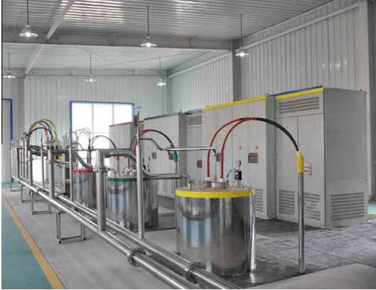
Fig. 1. SFCL in superconducting power substation.
